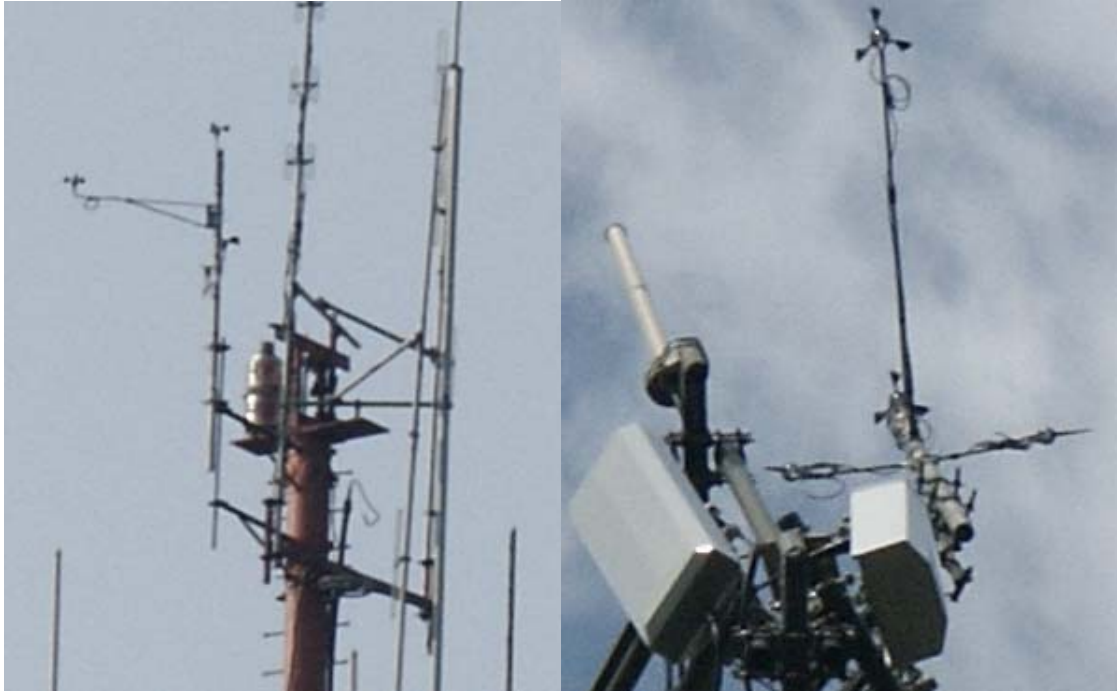
Figure 3-2. Paxton Tower Instrumentation.
